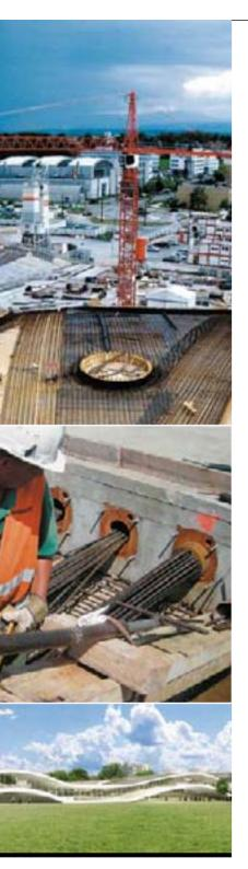
work, forming special concrete and developing a "hybrid static system", where some shells act as tied arches, while others bear on these arches while retaining their function as a shell.
