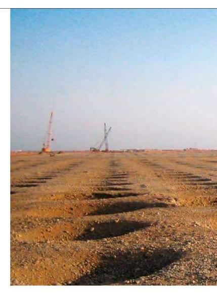
the work. "The presence of a shallow water table and the soil type meant that work also had to take place in various phases, representing up to five work phases for the same area, leaving the soil to rest between each phase," explains Armaud Meltz, project technical lead for Ménard.
