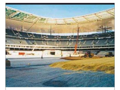
An alternate of the Menard Vacuum process, a venting system based on the use of drains and pumps and a waterproof membrane was installed under the Stade De France (St-Denis, France) to treat the gas fumes coming from the contamination of the ground. After working permanently for the first two years of operation of the stadium and allowing the extraction of some 500 tonnes of fuel, the system is now in operation for just one week per quarter.
