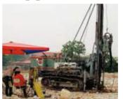
Malaysia. As a preliminary stage to constructing the east coast motorway linking the cities of Kuantan (in the South) and Kuala Trengganu (in the North), Menard Geosystems carried out soil improvement work over a 130,000 m<sup>2</sup> area. Two techniques were used: dynamic compacting and vertical drains linear metres).
