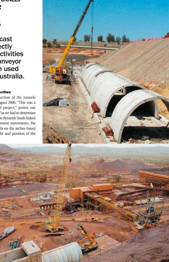
Two TechSpan arch tunnels have been built on the site of Mount Tom Price: one houses a receiving conveyor (see photo above) and the other an emergency exit.
