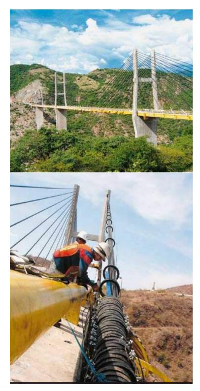
**B** UILT IN 1993 ON THE RIO DE LAS BALSAS, the Mezcala bridge is the largest structure on the Cuernavaca-Acapulco motorway and, due to its size and cablestaying, one of the most impressive in Mexico. The 882 m long bridge consists of six spans and its deck is supported by 140 stay cables, the upper sections of which are fixed to three pylons, the highest being 250 m, and arranged on six planes.
